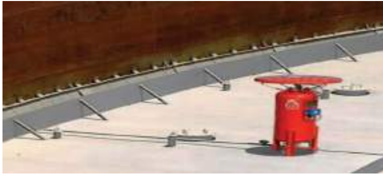
Fig.1.1 rim seal foam package system
