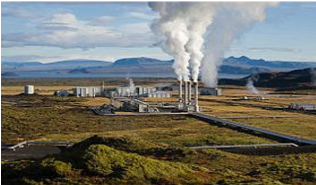
Steam rising from the Nesjavellir Geothermal Power Station in Iceland.
