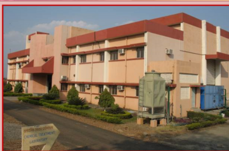
Main Building of Chemical Treatment Facility Lab
